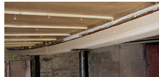
Apart from the improvement in airborne noise attenuation and fire protection, the Elasccon TCC system also distinctly improves bending strength and vibration resistance.
